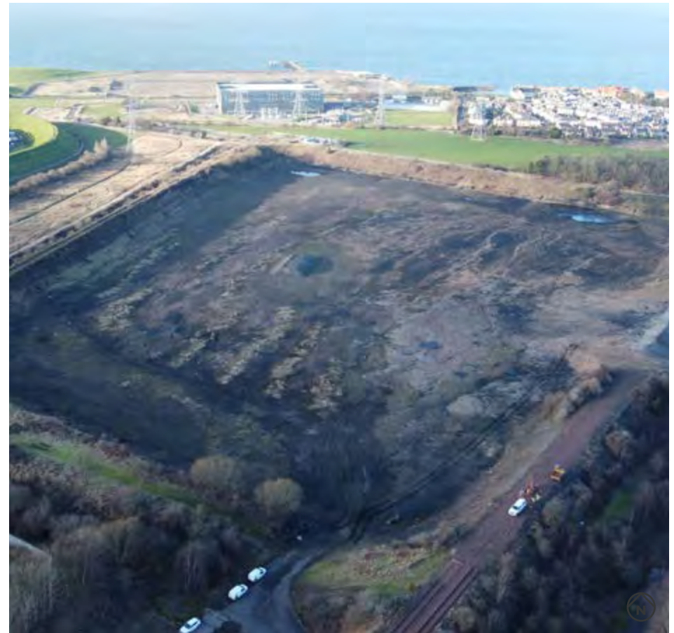
Figure 3- Coal Store Pre SLR Works
