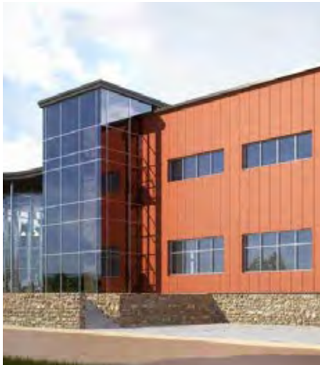
Stairtowers or vertical fenestration in elevations provides opportunities for changes in direction, and scale
