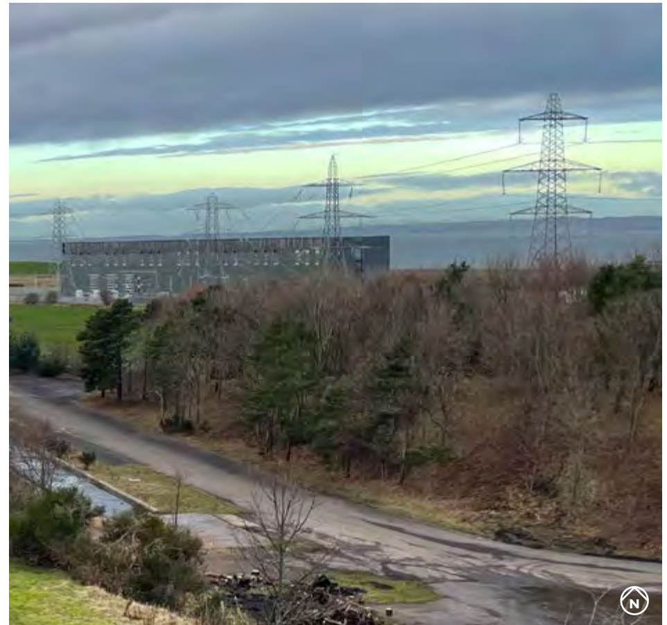
Figure 13- Existing Pylons on site
