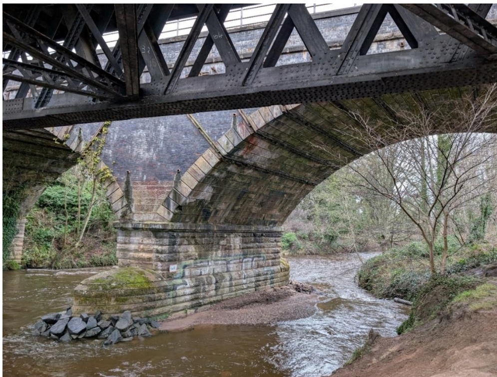
Figure A.44: Wooded and sharply incised valley of the River Esk, with walkway and river underneath the railway bridge
