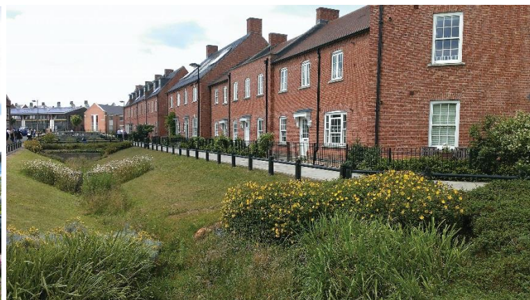
Figure 5: Examples of wet and dry planted swales. Source: The SuDS Manual C753
